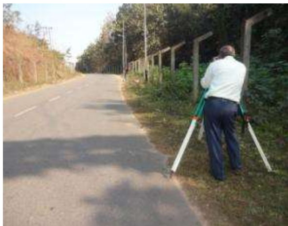
Photo 5: Raw water rising main alignment – survey going on
