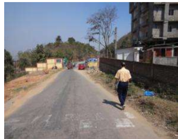
Photo 6: Raw water rising main near IOCL
